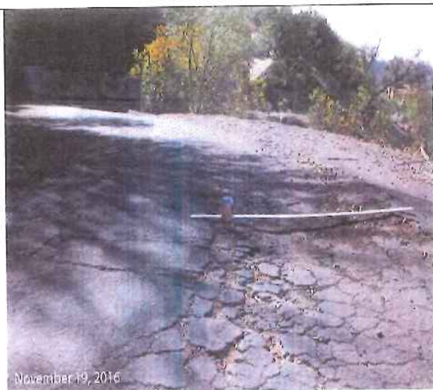
Exh. 2- Some of MWD Loop damaged-as of 2016 and it is worse today as no repairs have been made
